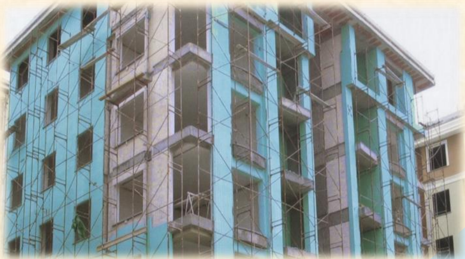
Figure 8: New rise building insulated with XPS (External Insulation)
