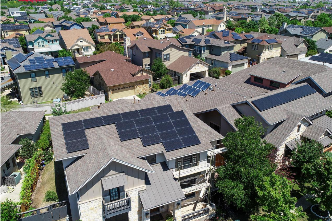
Figure 6 Private solar panels installed on roofs
