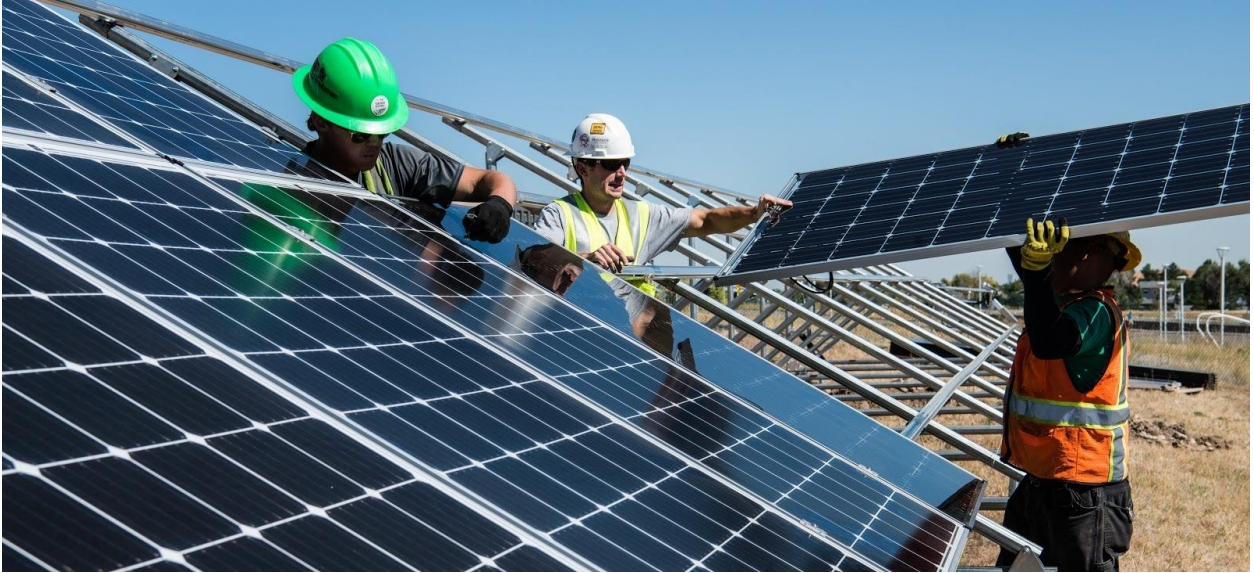
Figure 3 Solar panels installation
